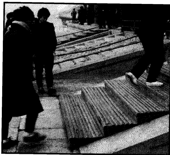
Figs 6.1 and 6.2 - The extraordinary hardness of bamboo cortex is utilized in China in the form of bamboo splints for covering the steps of wooden staircases to protecting them from wearing out, as can be seen in photographs 6.1 and 6.2. taken in the Forbidden City in Beijing, China, which is visited daily by thousands of tourists.
